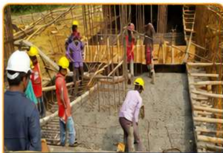
FOUNDATION & PILING WORK
