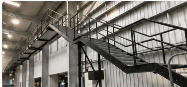
INDUSTRIAL MEZZANINE STAIRCASE
