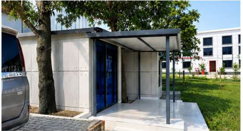
Project : Expo Accessories Ltd (MD Rest Room) Location: Salna, Gazipur, Dhaka.
