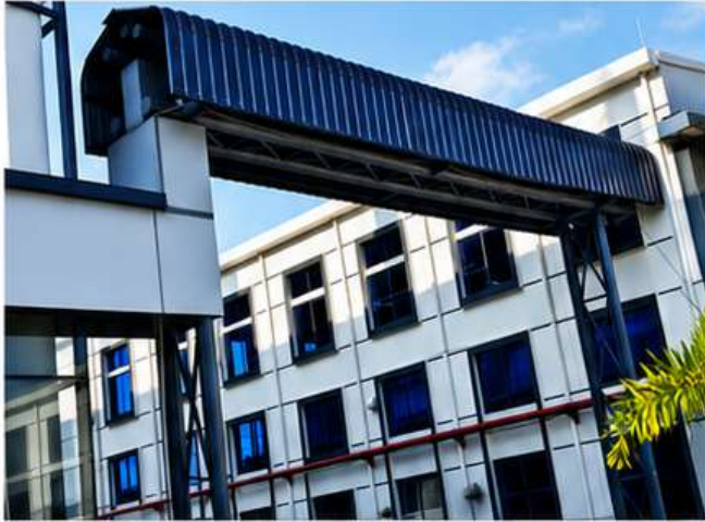
Project : Expo Accessories Ltd (BBT Bridge) Location: Salna, Gazipur, Dhaka.
