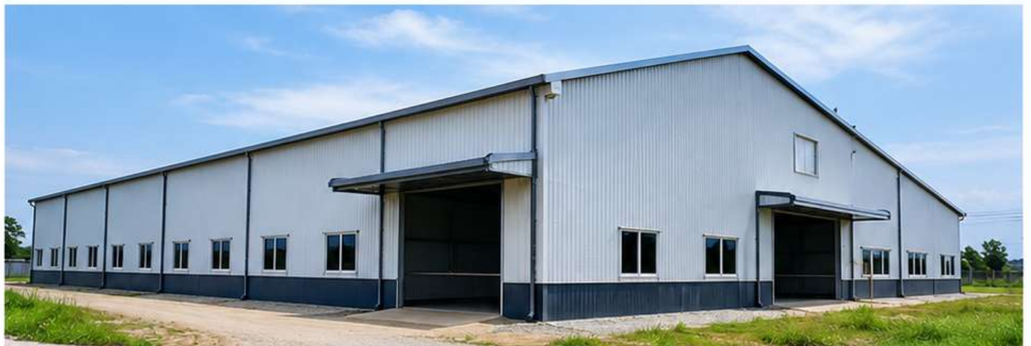
Project : Factory Shed Location: Nabinagor, Savar, Dhaka.
