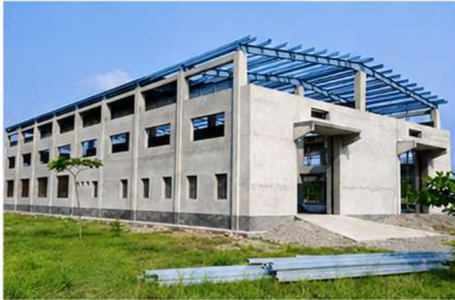
Project : Workshop Shed Location: BD Navy, Patuakhali.
