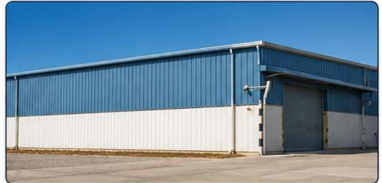
VERTICAL FASCIA WITH BACKUP PANEL AND VALLEY GUTTER
