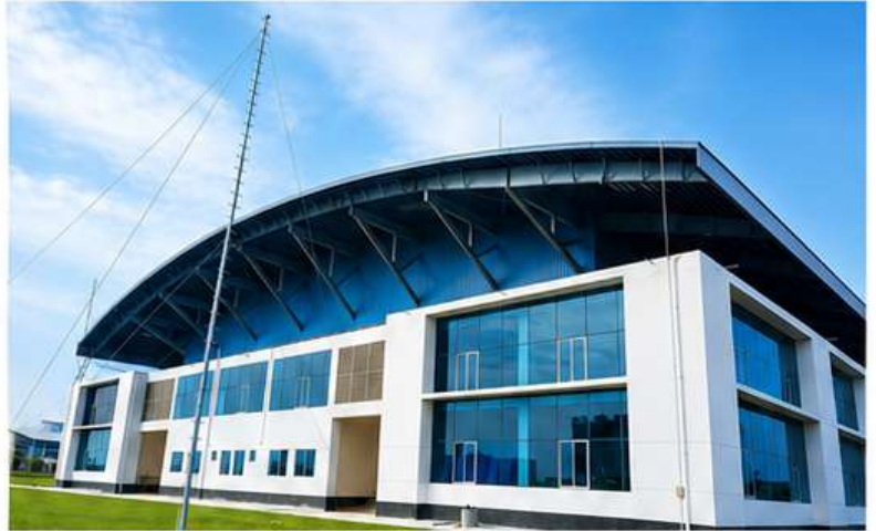
Project : Steel Shed Location: BD Navy, Patuakhali.
