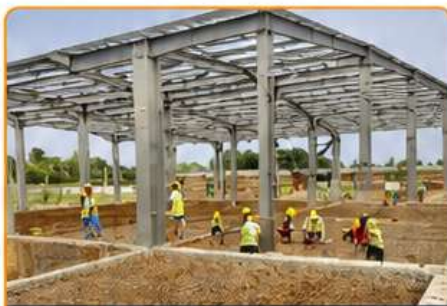
PEB & RCC CONSTRUCTION
